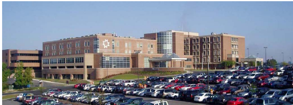
Photograph 2: Monongalia General Hospital from South-East, Exteriors Completed
