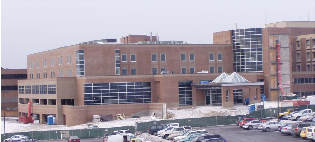
Photograph C 3: View from South-East showing the brick façade and curtain walls
